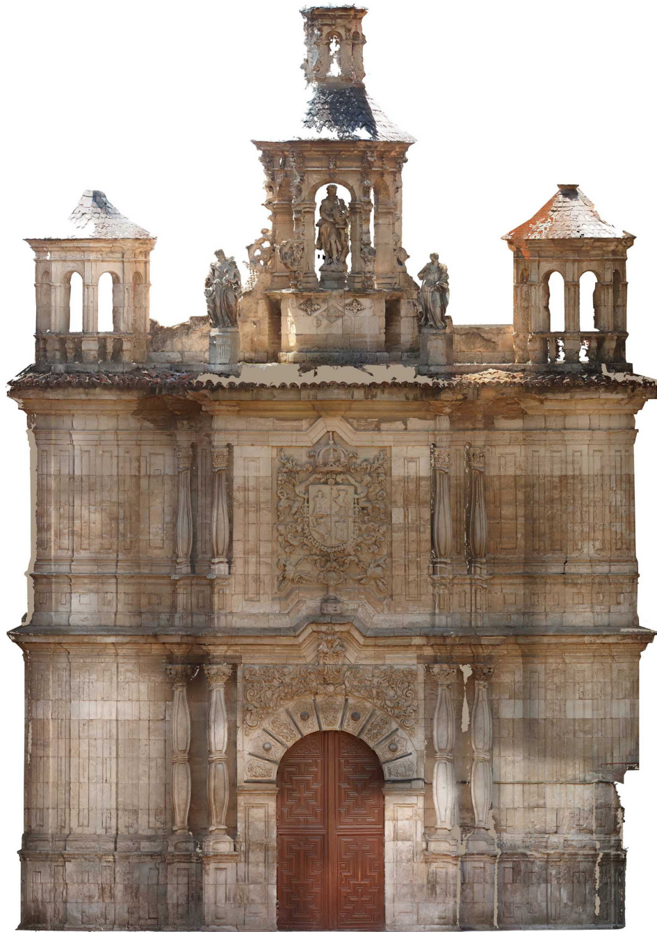
Figure 7. Texture and colour data of the façade of San Juan de Letran; example of compensated distortions of a photograph (Task Group's Partner: DAVAP Research Team , University of Valladolid, Spain).
