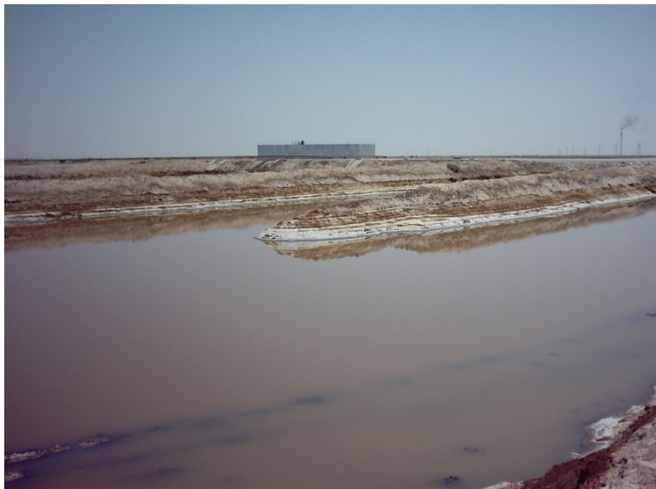
Figure 4. Mud pit condition after drilling operation.
