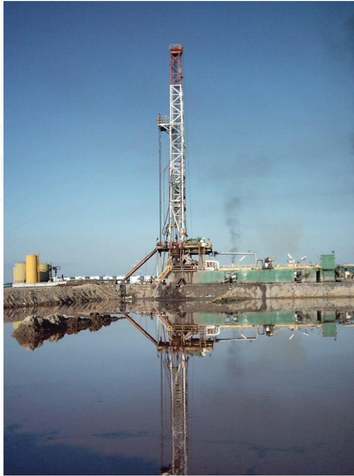
Figure 3. Mud pit condition during drilling operation.
