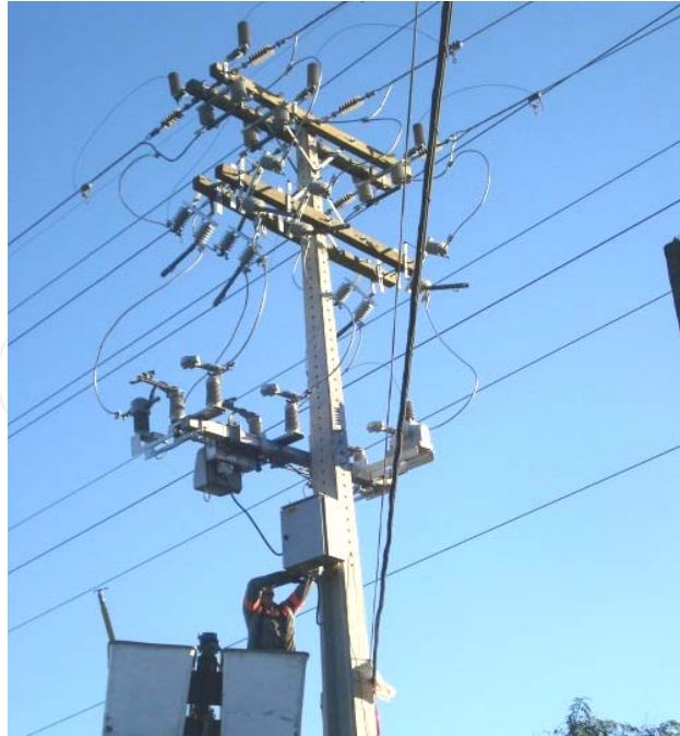
Fig. 8. Installation of a remote controlled switch.
