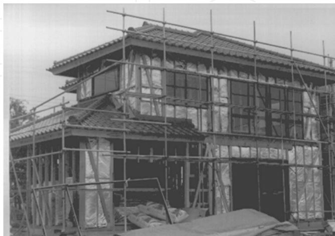
Figure 1. Common wooden structure of Japanese house under construction
