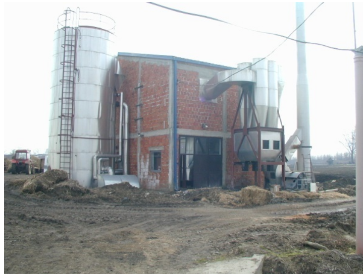
Figure 18. The boiler house, heat accumulator and cyclone type separator
