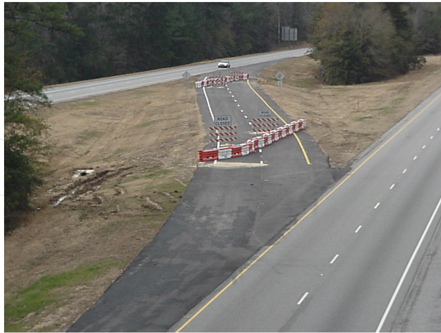
Figure 2. Traffic control using temporary barriers during contraflow operations
