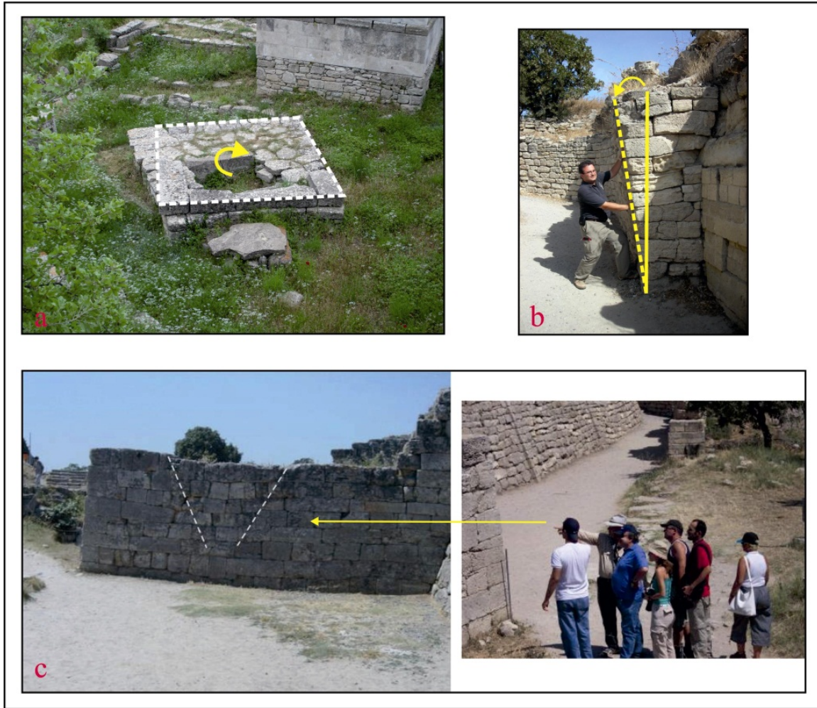
Figure 2. Deformation structures of seismic origin within Troy VI Layer a) clockwise rotation b) Tilting c) systematic cracks in the walls of Troy VI Layer that Prof. Manfred Korfman showed the project team
