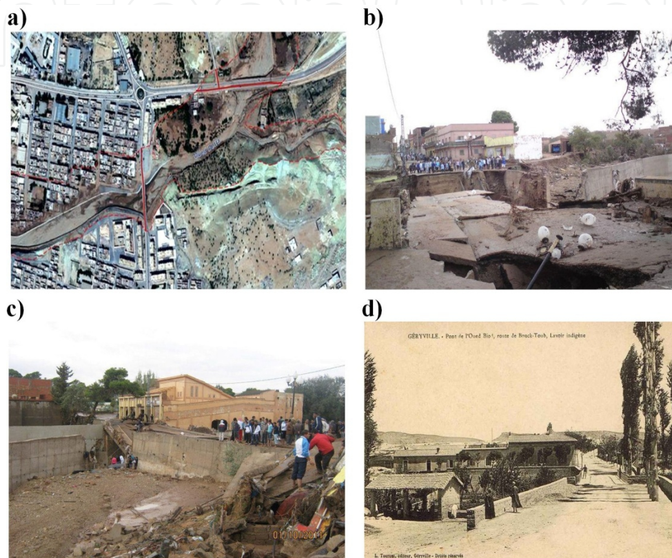
Figure 3. Impact of flooding – El Bayadh City on October 01, 2011. a) Satellite images, Algerian Alsat-2A [ASAL, 2011], b), c) and d) Destruction of the Historical Mahboula Bridge.
