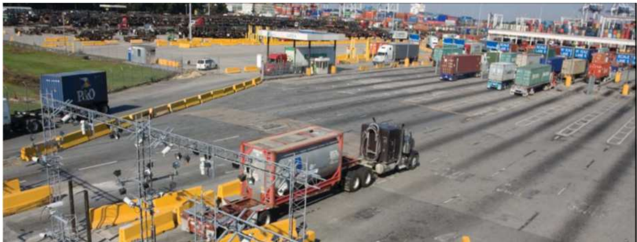
Fig. 12. Reading infrastructures OCR/RFID in Georgia Port Authority. Courtesy of Identec.
