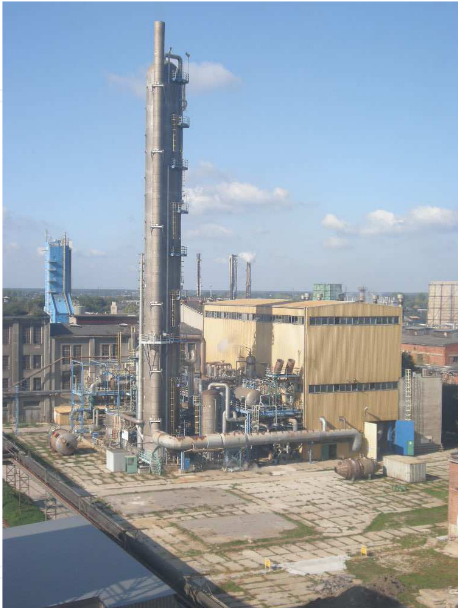
Fig. 1. Nitric acid plant in AZOTY Tarnów
