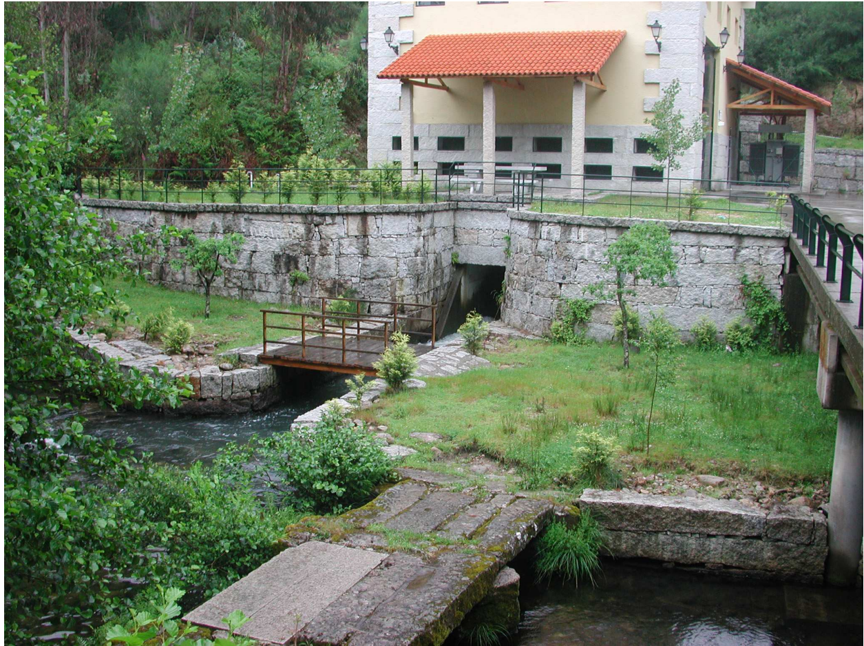
Fig. 2. Central power station of the DevaPO River (Pontevedra, NW Spain).
