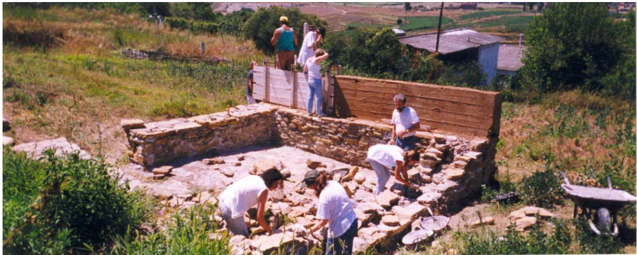
Fig. 12. Building the experimental granary at l'Esquerda in 1998, with P.J. Reynolds standing near the adobe wall
