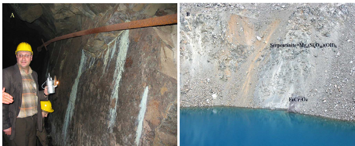
Fig. 6. Seepage waters from surface to deep (A) in the gallery; serpentinite and chromitite (B).
