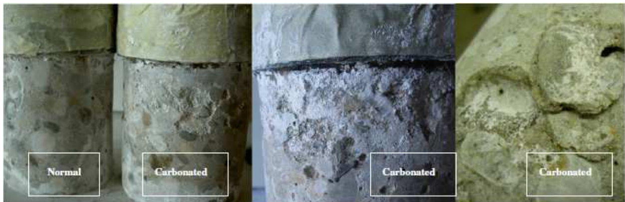
Fig. 17. Visual observation of normal and carbonated concrete specimens exposed to sodium sulfate solution [53]
