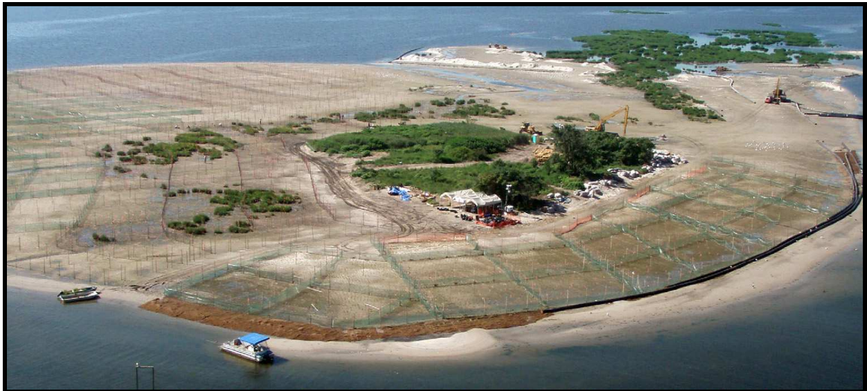
Fig. 6. Construction of Elders Point West July 2010.
