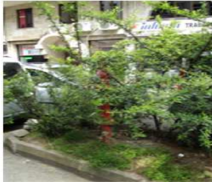
Fig. 5. Example of the lack of visibility of some hydrants covered by plan (Nisanci, 2010).
