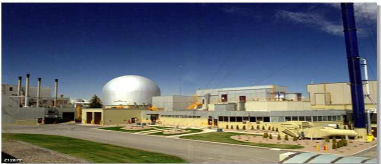
Fig. 1. Fuel Conditioning Facility.
