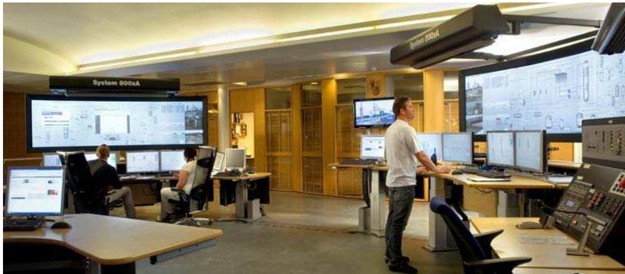
Fig. 5. Extended Operator Workplace from ABB with interactive large display.
