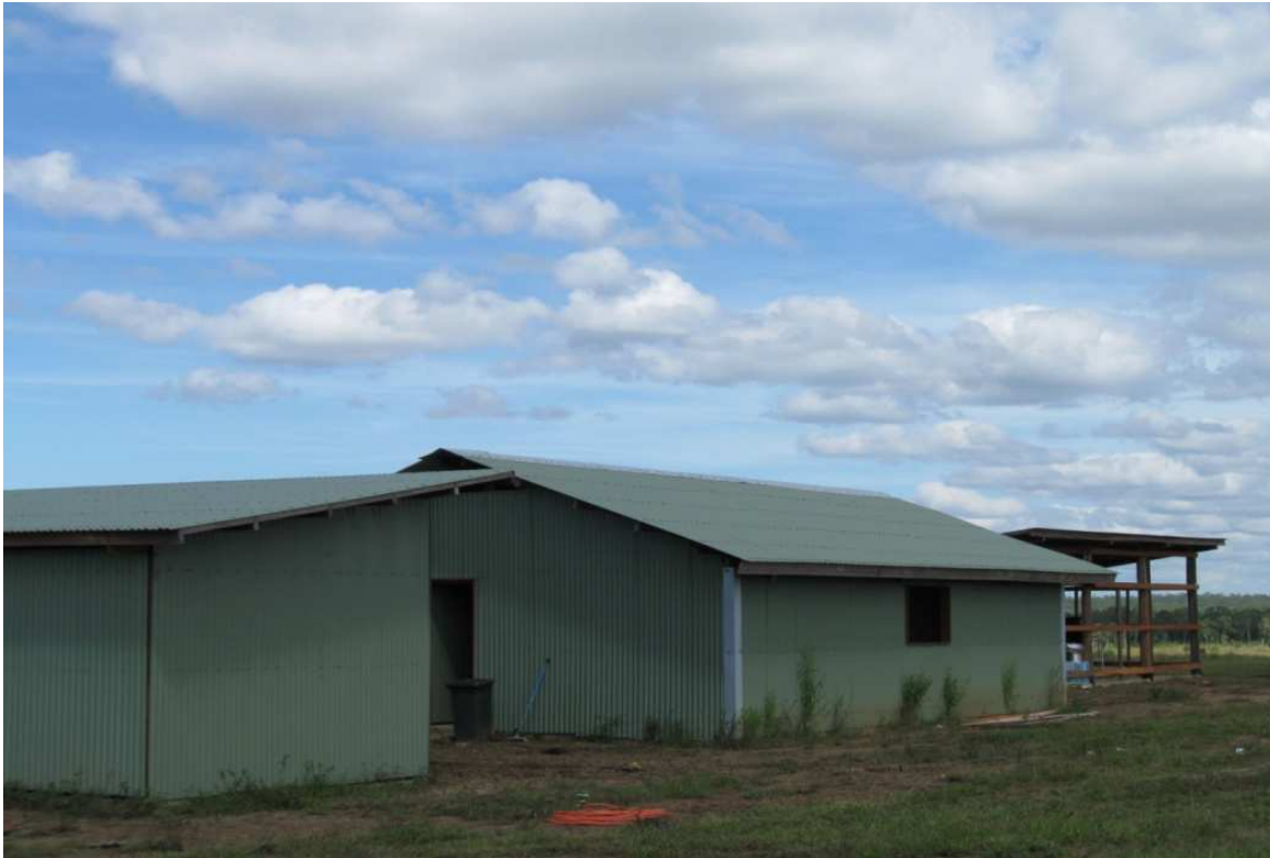
Fig. 3. The Garrathiya Dormitory and Outbuildings during Construction
