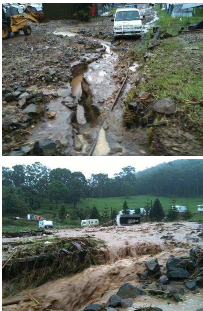
Fig. 1. Woodfordia Storm Damage – January 2011.
