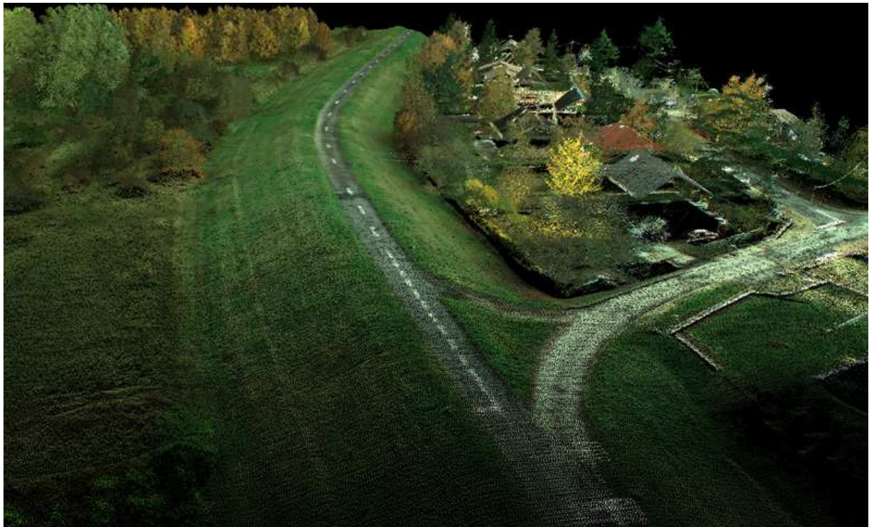
Fig. 5. Colored 3D point cloud over a dike (source FloodProBE - FUGRO)
