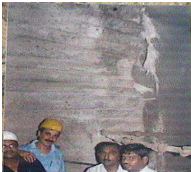
Fig. 5(b). Pier nose wall after pre-split blasting
