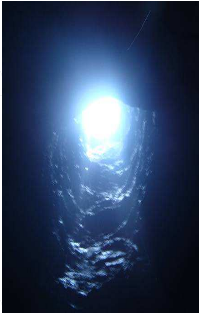
Fig. 4. Profile of pilot surge shaft excavated by long hole raise driving at Koilsagar
