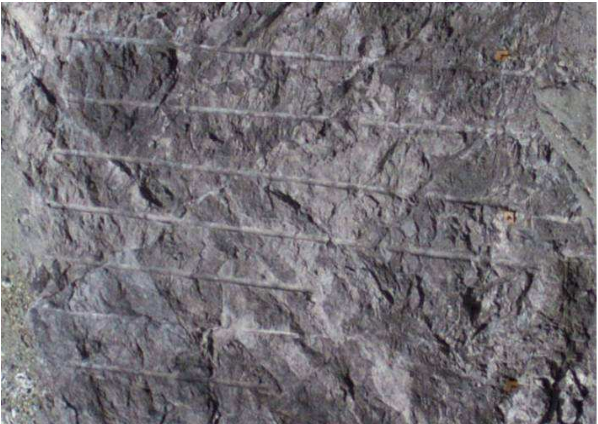
Fig. 7. Improved blast performance of smooth blasting in the form of smooth profile at KHEPP
