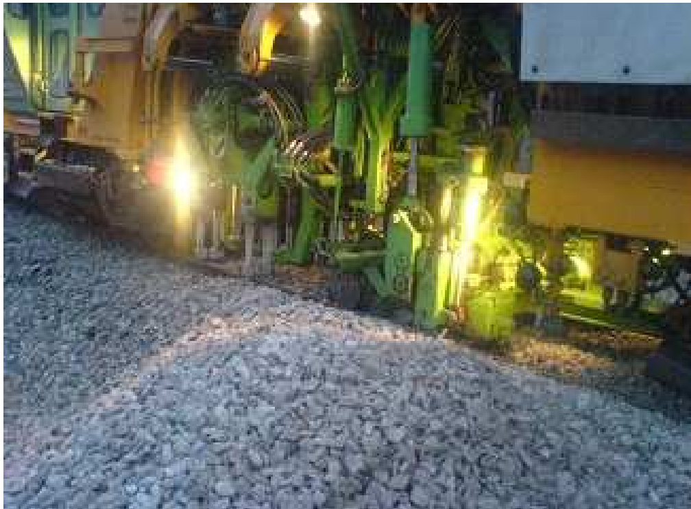
Fig. 17. Tamping and stabilizing operations after the installation of the railway track with B70-F sleepers (before the second stage of test)
