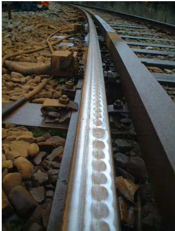
Fig. 2. Example of rail corrugation
