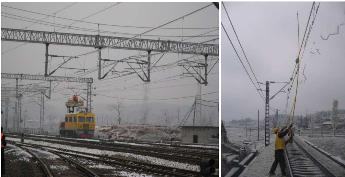
Fig. 1-1. Manual de-icing on overhead contact wires
