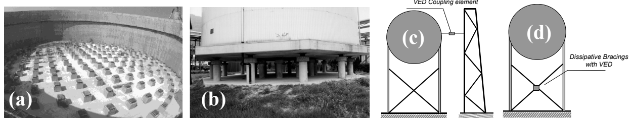
Fig. 10. a) Base isolation of a LNG tank at Revythousa Island (Greece), b) Base isolation of an elevated tank ammoniac tanks at Visp, Switzerland, c) Dissipative bracings solution for elevated tanks, d) dissipative coupling solution for elevated tanks.
