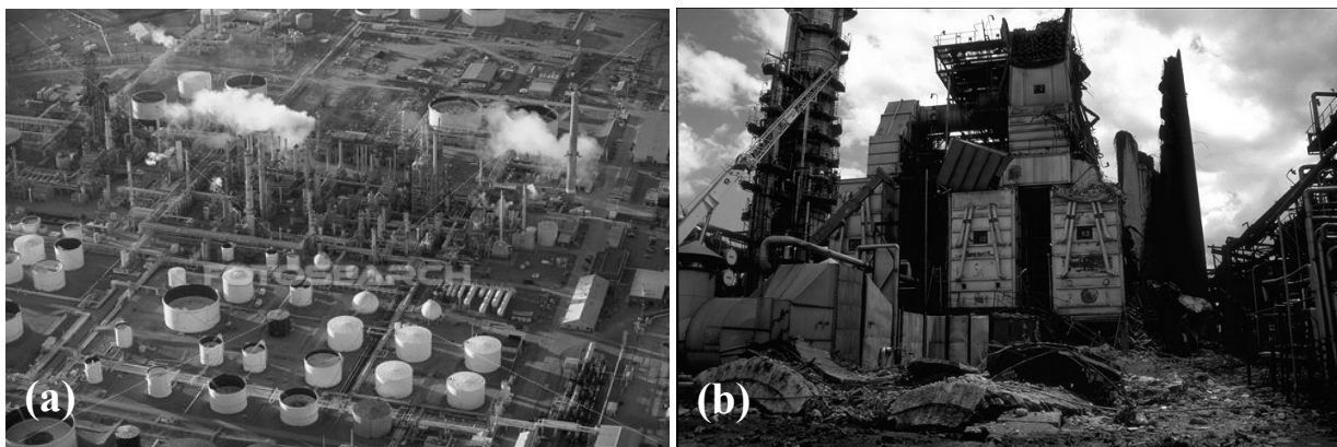
Fig. 1. (a) Areal view of a refinery, (b) Damage in a process furnace (Izmit, 1999).
