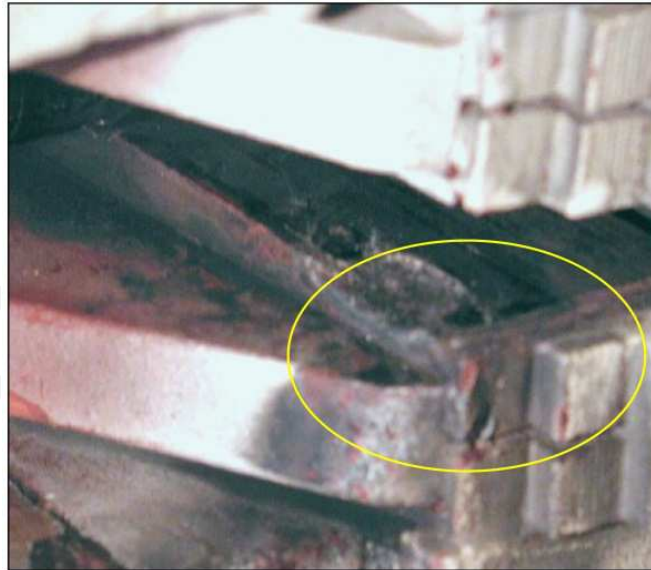
Fig. 3.5.1.2. Damages evidences in the stator core laminations of TG-2.
