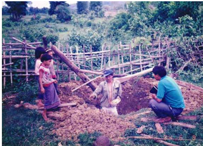
Picture 3. Making of pit for toilet
