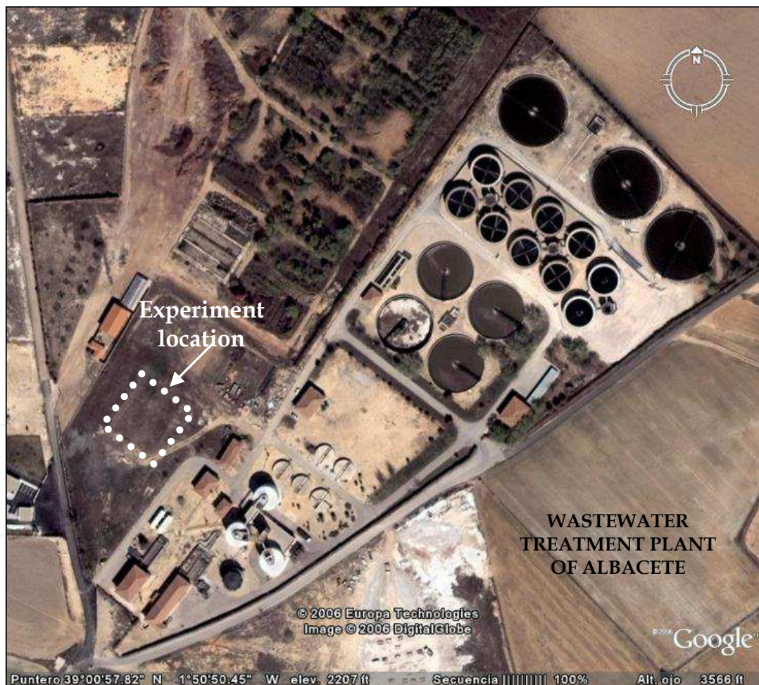
Fig. 1. Location of the experiment in the wastewater treatment plant of Albacete
