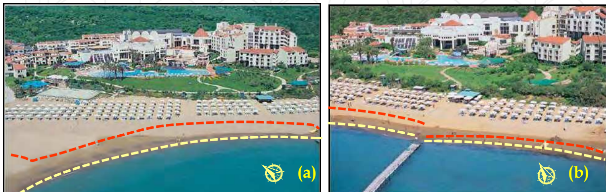
Fig. 8. Perissia Hotel Beach at Side; shoreline retreat due to erosion over the years, red line shows the shoreline position approximately in August, 2006 (a: view of the western part of the beach from sea, b: view of the eastern part of the beach from sea; pictures from 1999; Güler et al., 2008)
