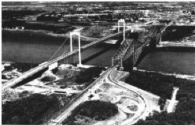
Fig. 6. Iron bridge arc-sprayed with zinc and then painted Ducos (2006) .
