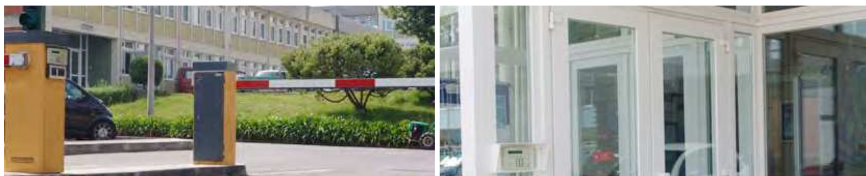
Fig. 7. Campus Access control - Instituto Superior de Engenharia de Coimbra . Installed car park and building access, by a security contractor using HID RFID technology.
