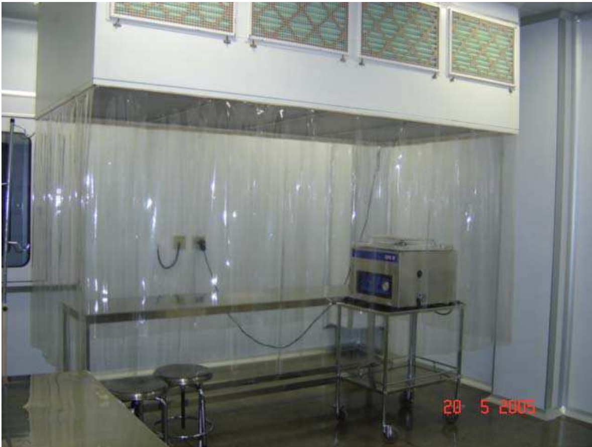
Illustration 03. Classified processing room (100 particles/m 3 air: Class 100/ISO 5; HEPA Filters 99.9 %)
