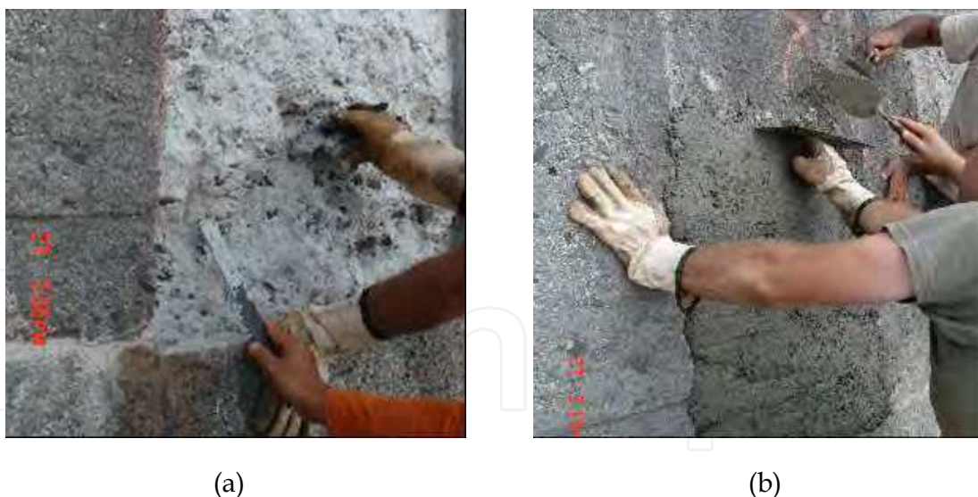
Fig. 10. (a) Application of bridge bonding. (b) Launch of the repair material.
