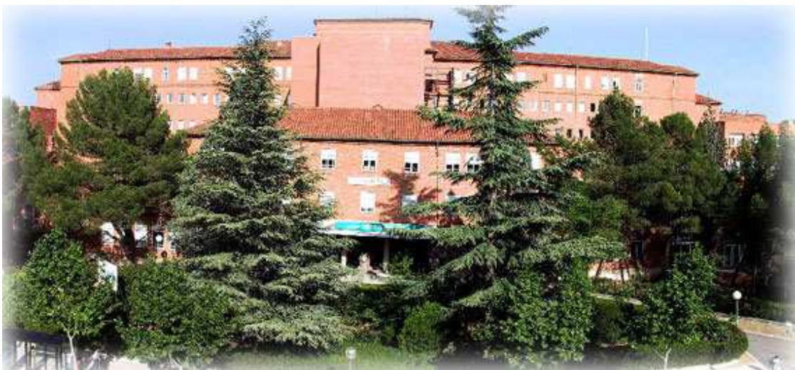
Fig. 9. Hospital Obispo Polanco, inaugurated in 1953. Teruel, Spain
