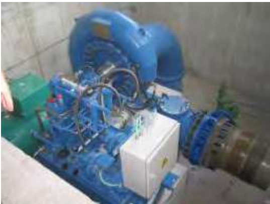
Photo 25. Francis turbine with a spiral casing (case study Sangüesa).
