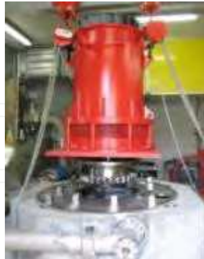
Photo 8. Le Châble Profray: The turbine and its runner and the alternator, during the erection.
