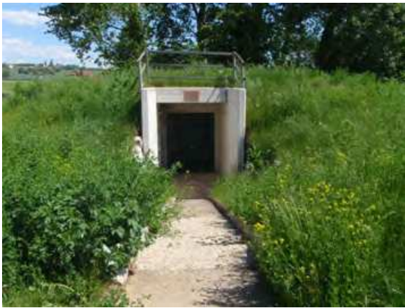
Photo 3. Armary: the power house.
