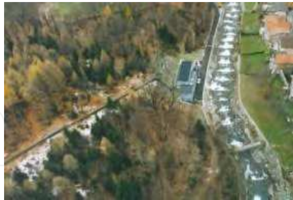
Photo 6. Rino: a view of the power station.
