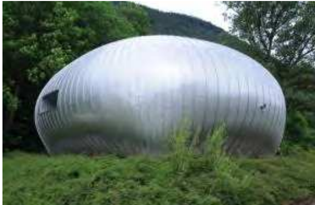
Photo 9. Seefeld: the power house.
