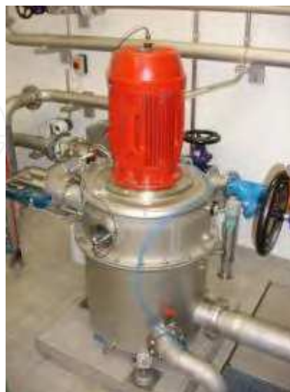
Photo 33. Counter pressure Pelton turbine (Fällanden SHP plant, Switzerland, set in a drinking water network, H = 140 m, Q = 16 l/s, P = 17 kW, 2008).
