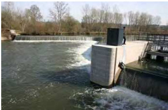
Photo 19. L'Ame: downstream global view of the dam and the turbine.
