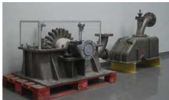
Photo 22. Tordera: a dismantled Pelton turbine.
