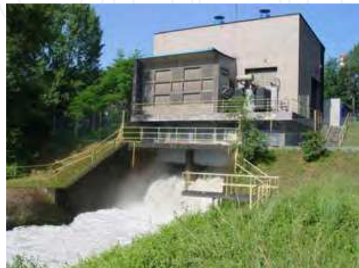
Photo 24. Skawina: the powerhouse during turbine overhaul.
