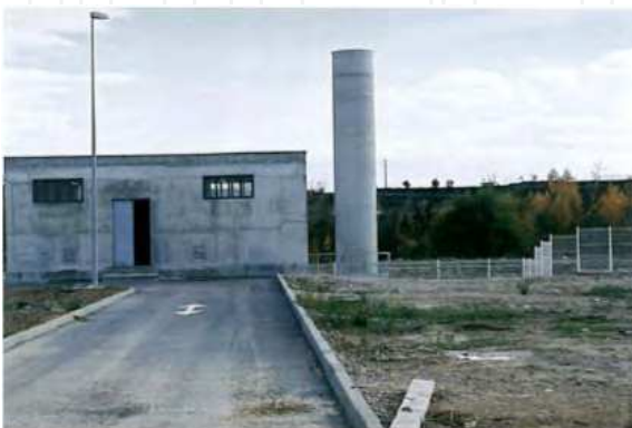
Photo 23. Sangüesa: the biomass plant and its tower of 10.5 meters.
