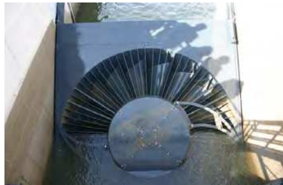
Photo 20. L'Ame: upstream view of the turbine.
