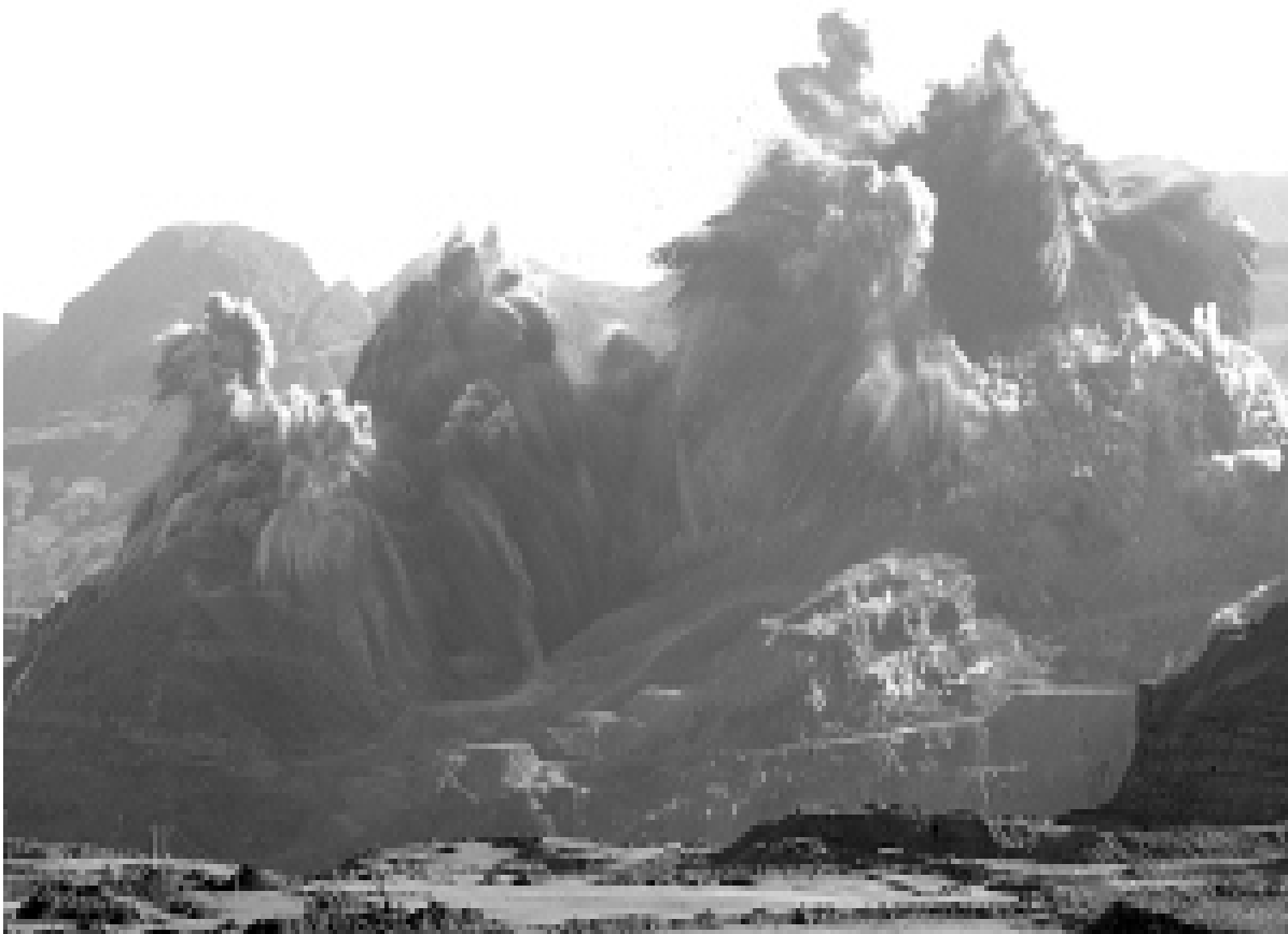
Fig. 7. Throw blasting in Dafeng mine.
