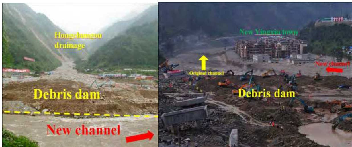
Fig. 25. The blocked Ming River and new Yingxiu town in flood by Hongchungou debris flow.
