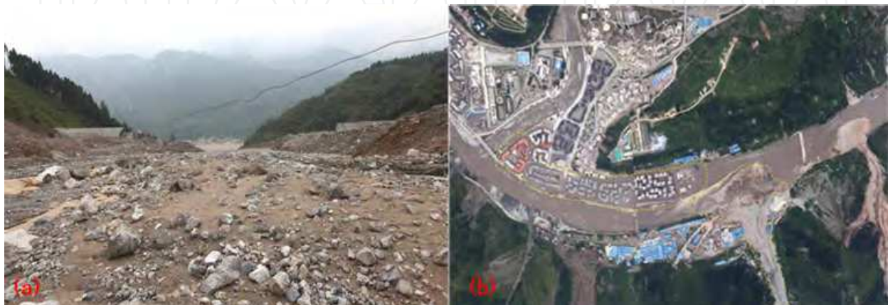
Fig. 23. (a): The destroyed check dam in Qingping debris flow; (b): Ming river blocked at Yingxiu town by Hongchungou debris flow ( photographs from Tang chuan)
