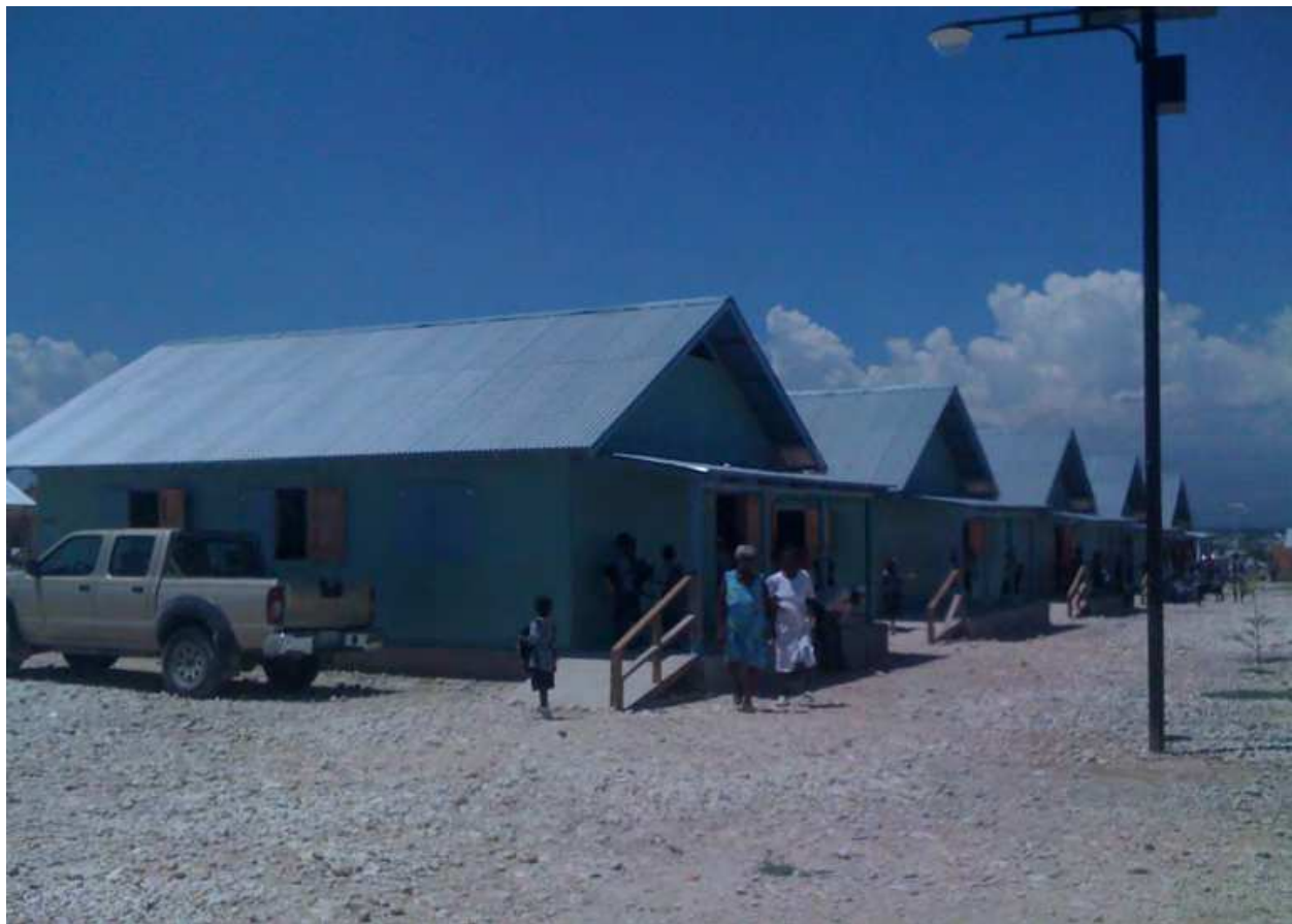
Fig. 7. New classroom buildings with ramps (Camp Corail, Croix-des-Mission, Haiti).
