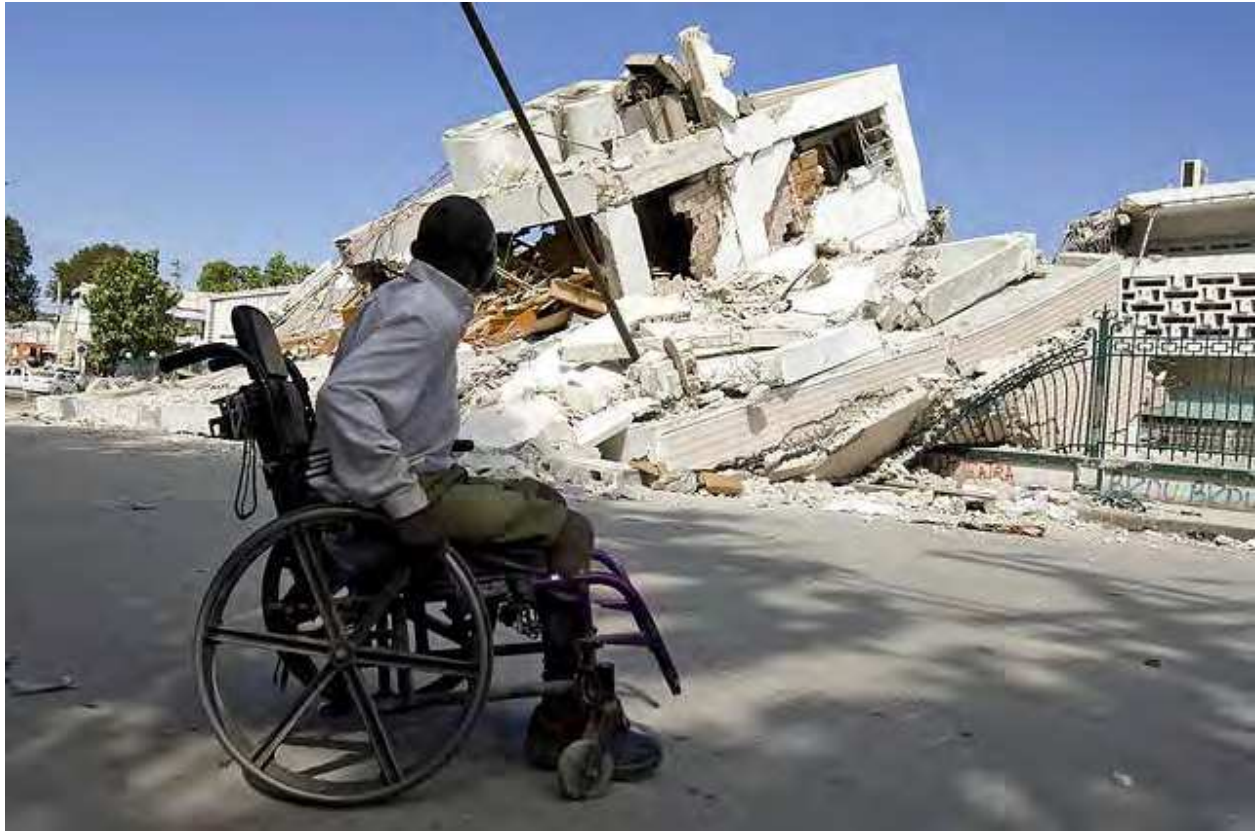
Fig. 4. The earthquake in Haiti caused significant damage to buildings in Port-au-Prince (UN, 2010)
