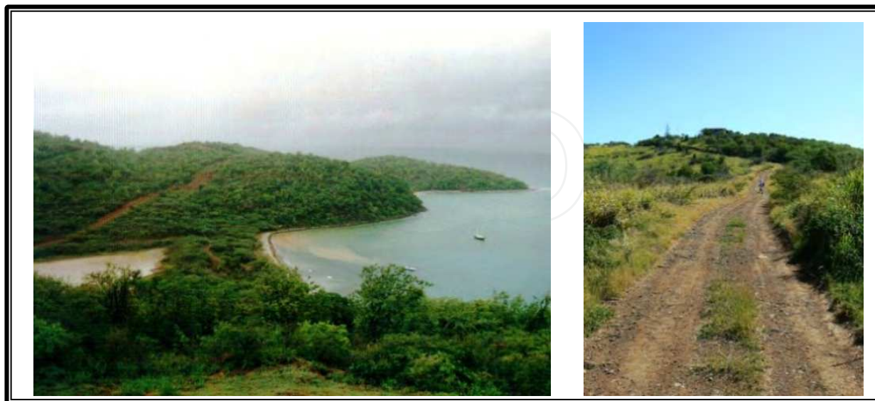
Fig. 2. (Left) Picture of a plume entering Bahía Mosquito by sediment produced from a single, unpaved road segment (photo courtesy of M.A. Lucking-CORALations). (Right) Picture of an unpaved road segment that typifies the road network in Culebra.
