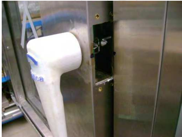
Fig. 9. New lock assembled for a test
