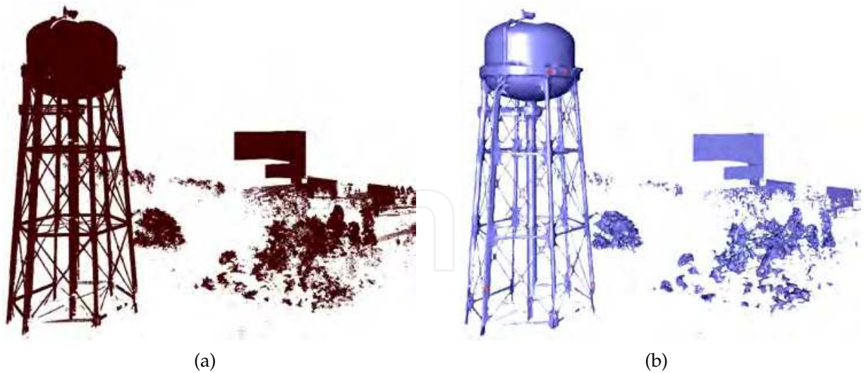
Fig. 10. Water tower scan at the campus of UC Davis. (a) Raw point cloud having 4.3 mio. points, (b) reconstruction having 300k faces (10 subdivision steps) (total reconstruction time of about 23 seconds performed with an Intel Core2 Duo).
