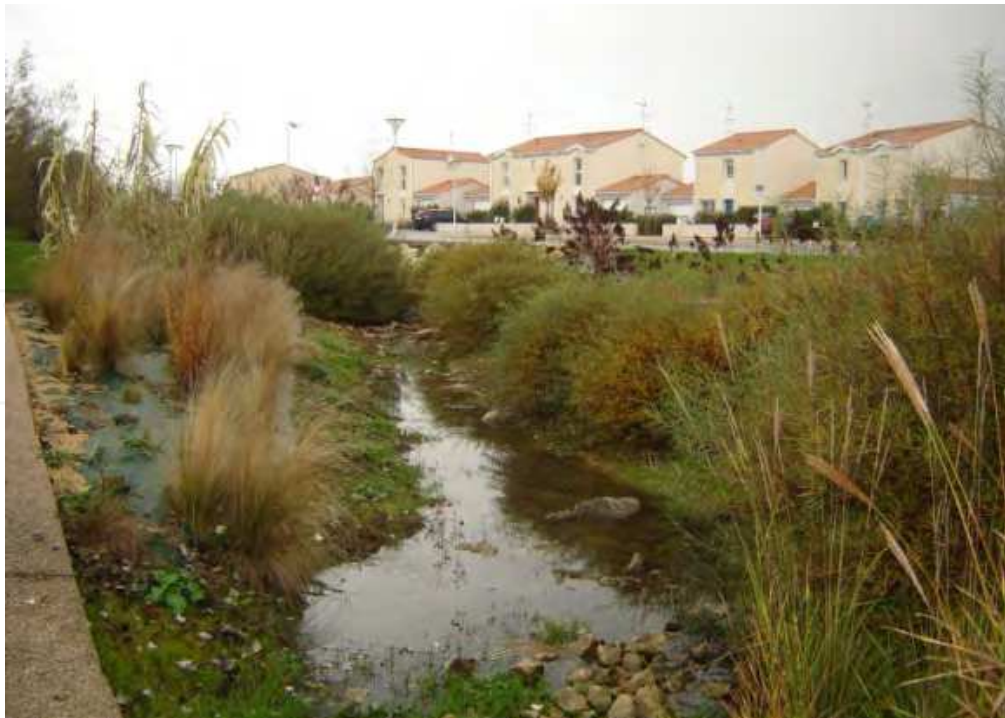
Fig. 5. A retention pond in Lagord, France (Photo Rezende, 2009).
