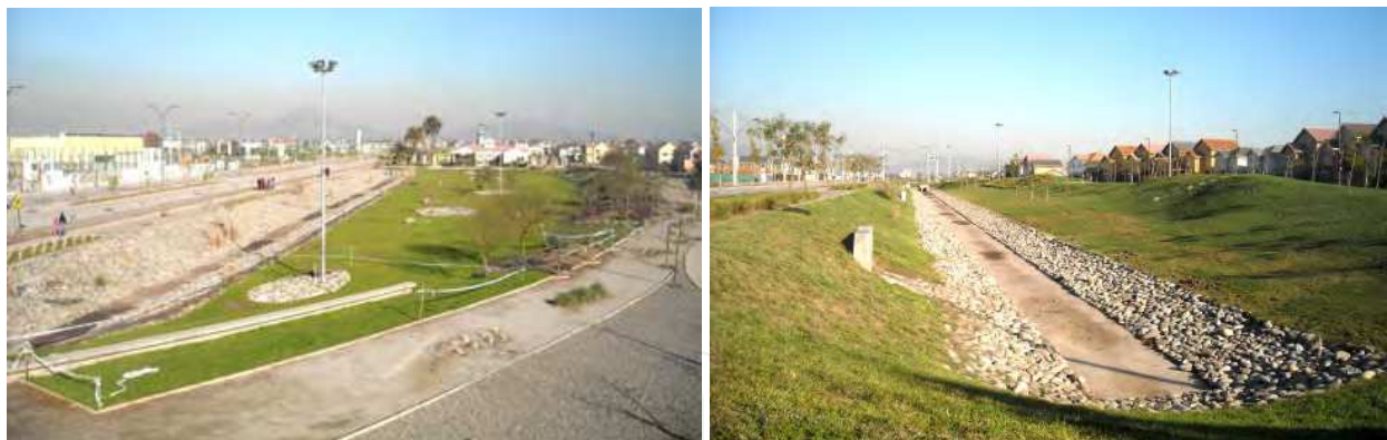
Fig. 4. A detention pond in Santiago, Chile (Photo Miguez, 2009).
