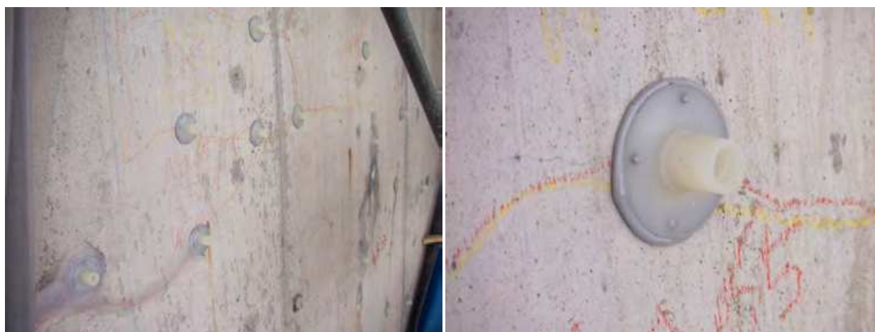
Fig. 1. (a) Multiple locations of injection on the surface, (b) detail of the injection point.
