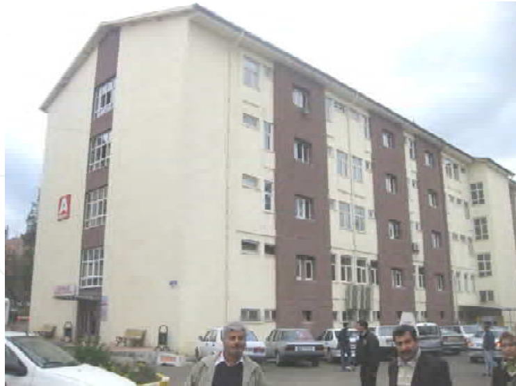
Fig. 8. An external shear wall strengthened building
