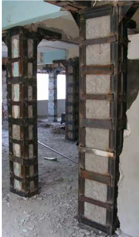
Fig. 13. Steel jacking applied to RC columns (Photo by Dr. Ali Haydar Kayhan)
