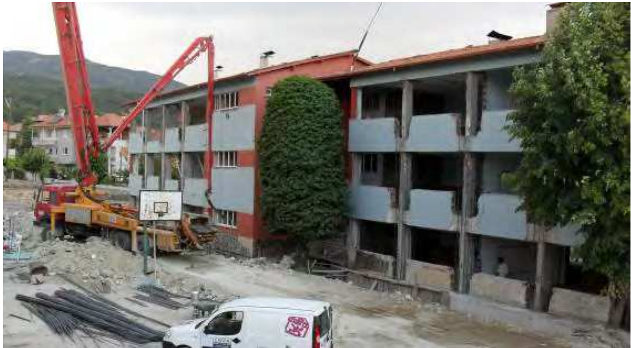
Fig. 12. An RC jacketing application (Photo by Ahmet Sarışın)
