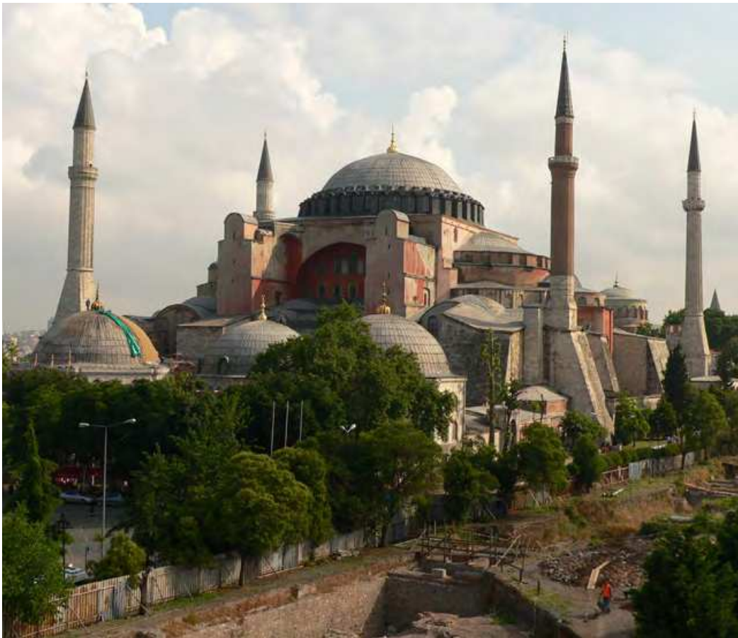
Fig. 1. Hagia Sophia is strengthened with external buttress type walls by Sinan in 1573.
