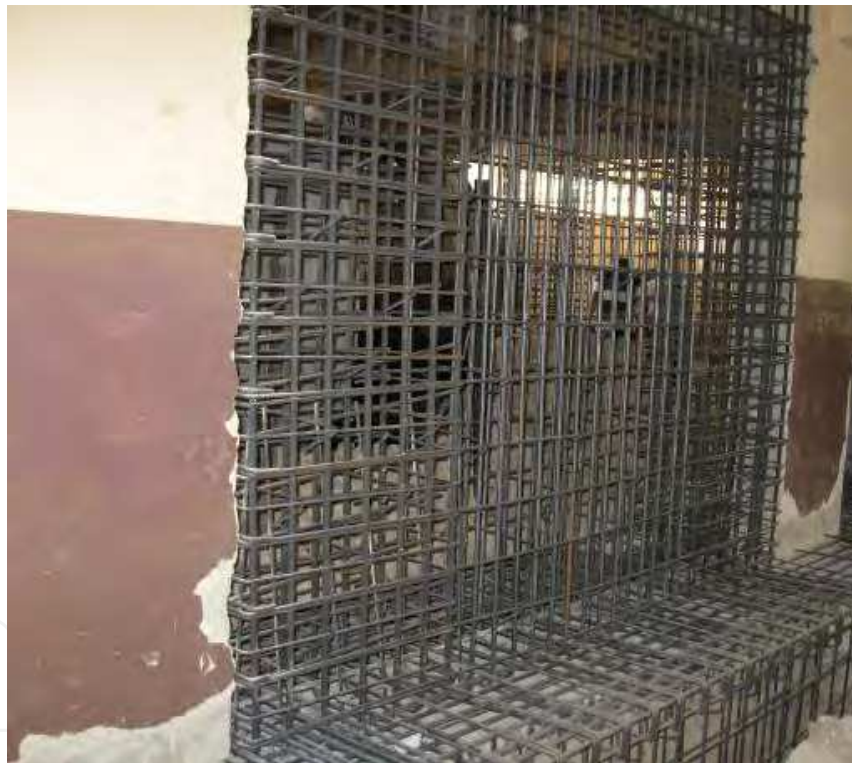
Fig. 3. Infill wall application in an RC building
