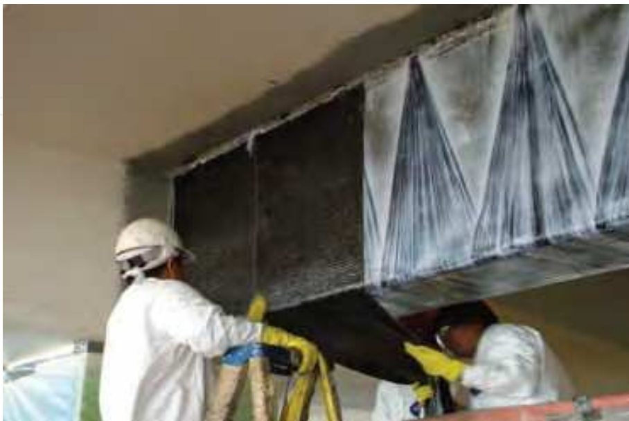
Fig. 14. FRP confinement of a beam (reprinted with the permission of FYFE Europe)
