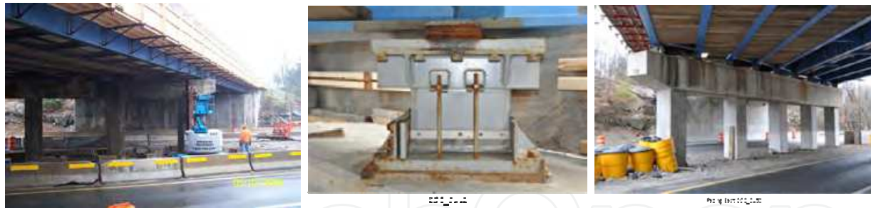
Two Span Bridge Rehabilitation Roller Isolation Bearing Installation at Completion
