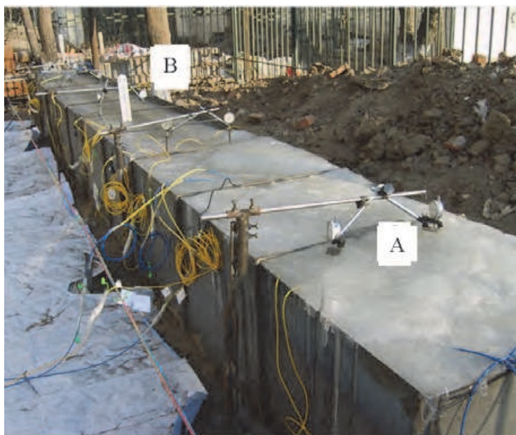
Fig. 39. Profile of frost-heaving
