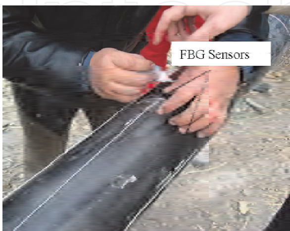
Fig. 44. FBG sensor installation
