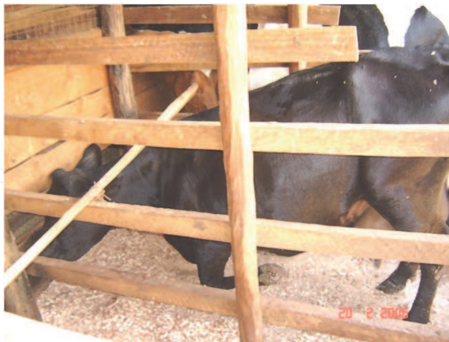
Fig. 18. Inadequate lunging space and bob zone causing difficulties for the cow during standing due to low cross-bar in the cubicle and short length of the cubicle. These were found in some of the zero-grazing units during the study of prevalence and risk factors of claw lesions in the peri-urban areas of Nairobi, Kenya.
