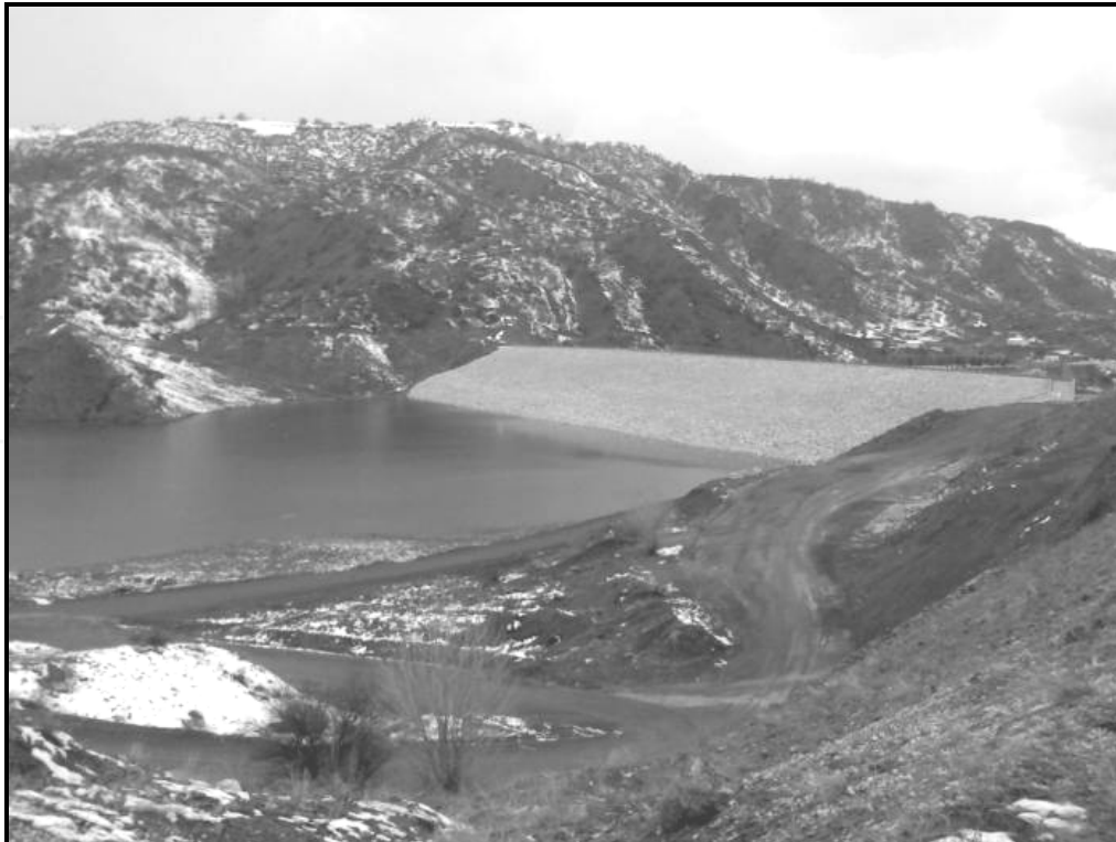
Fig. 9. View of the Hatap dam
