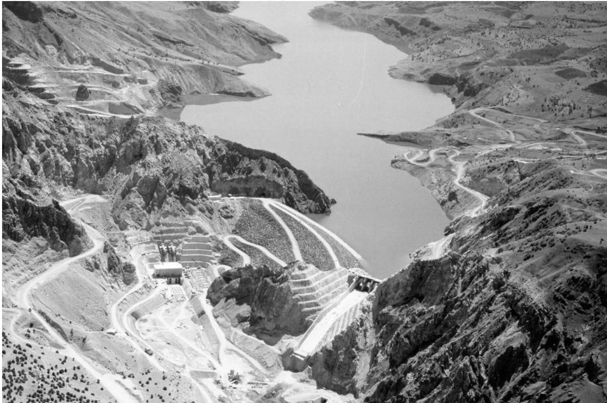
Fig. 7. View of the Kilickaya dam
