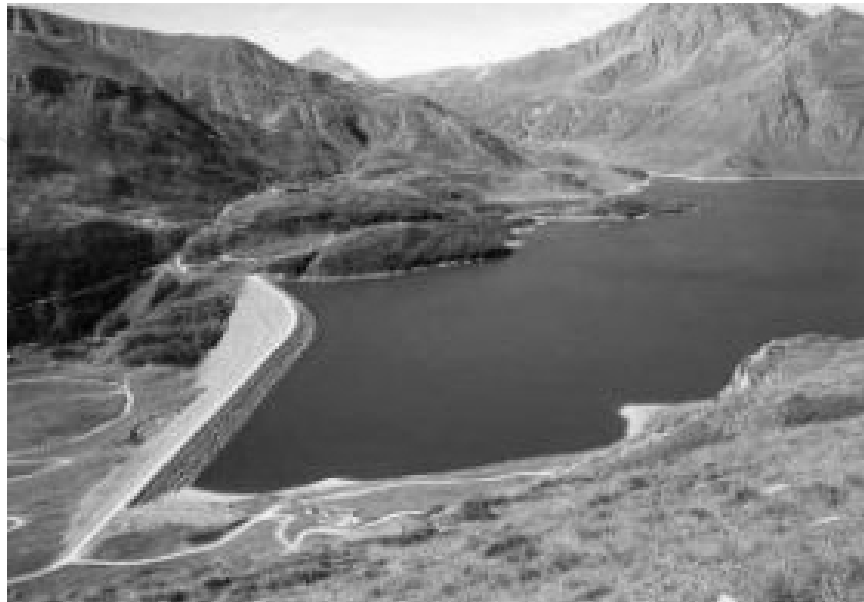
Fig. 13. View of the Boztepe dam
