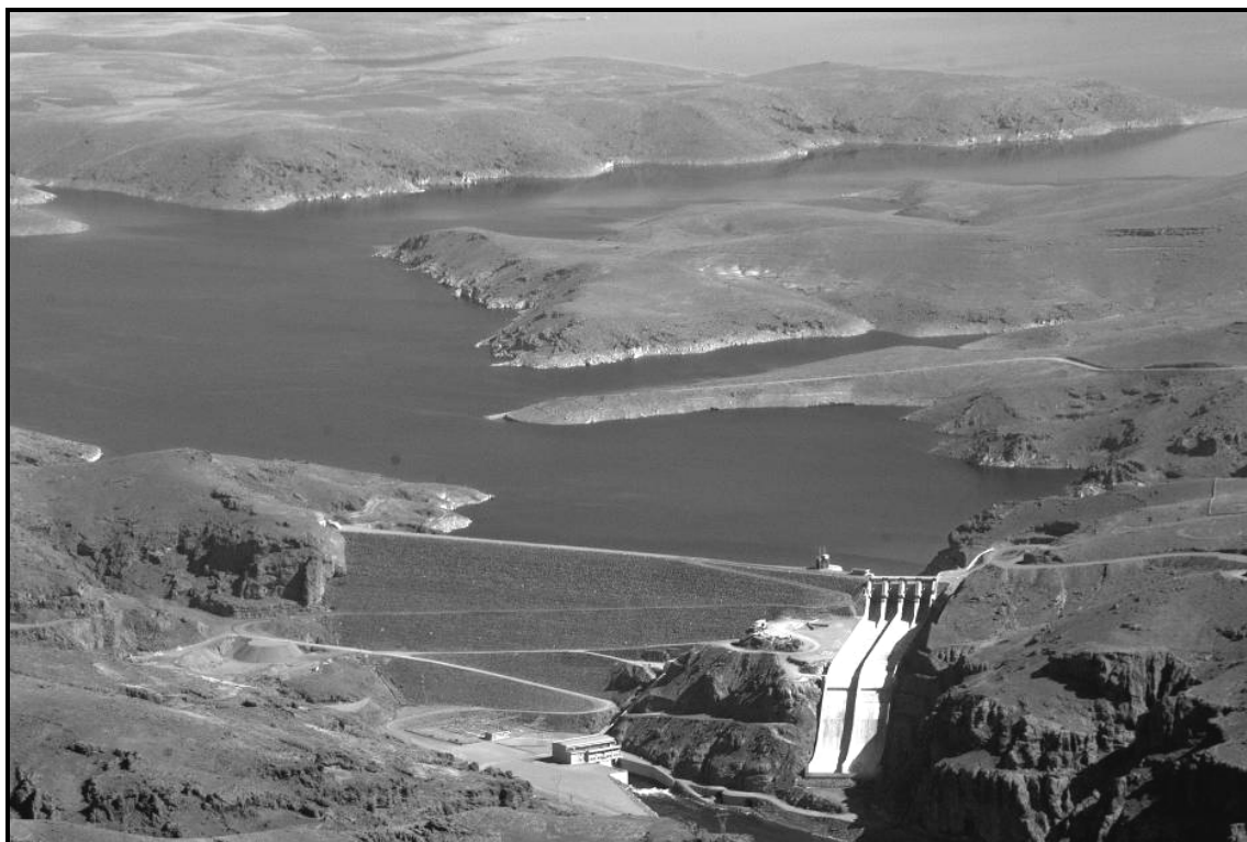
Fig. 11. View of the Ayhanlar dam
