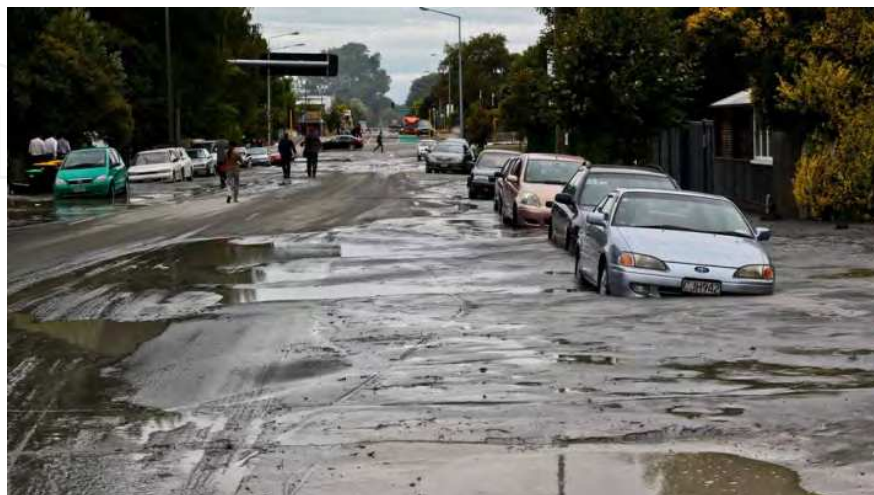
Fig. 26. Liquefied Sand Deposited on Street, 2011. http://otilya.com/view/News/Asia-Pacific/New-Zealand
