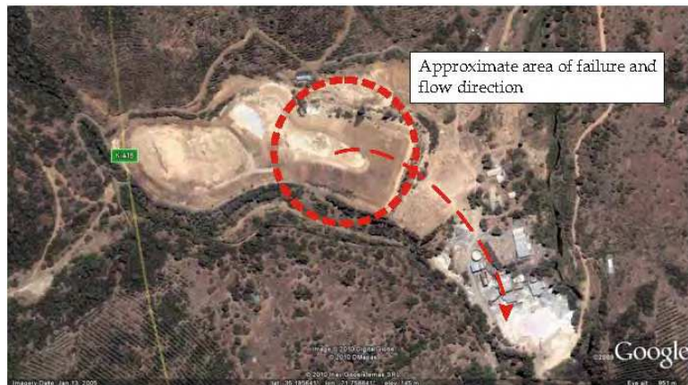
Fig. 23. Bird's-eye View of Las Palmas Tailings Impoundment Prior to Failure. (GEER 2010)
