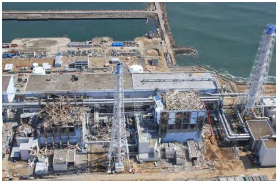
Fig. 34. Blast-Damaged Fukushima Dai-Ichi Nuclear Power Plant Unit 3 (left) and Unit 4 (right). http://pinktentacle.com/
