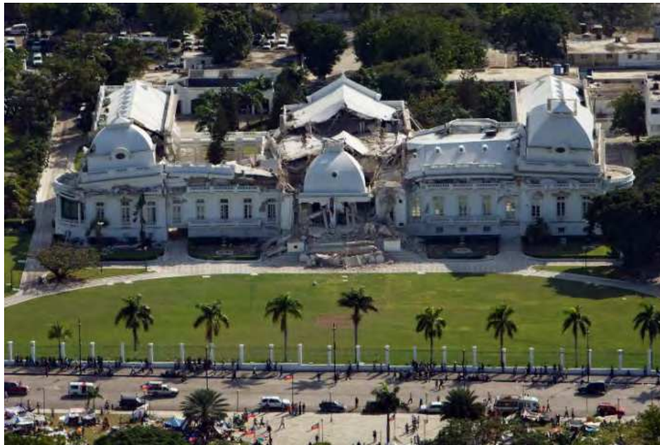
Fig. 20. Damaged Presidential Palace in Port-au-Prince. http://alanrdennis.wordpress.com
