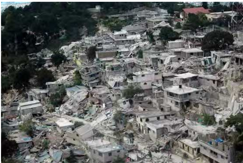
Fig. 19. Damaged Buildings Located on Hill Slope. http://www.worldcatastrophe.com
