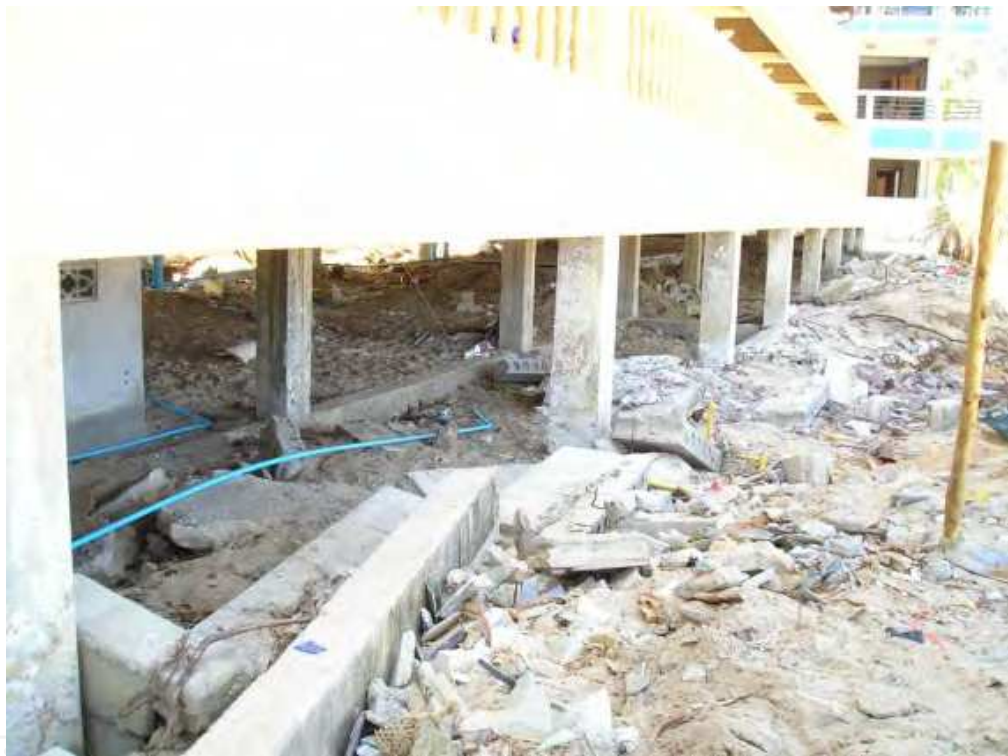
Fig. 42. Close-up of Fig. 41, Showing Inter-connected Grade Beams and Columns.
