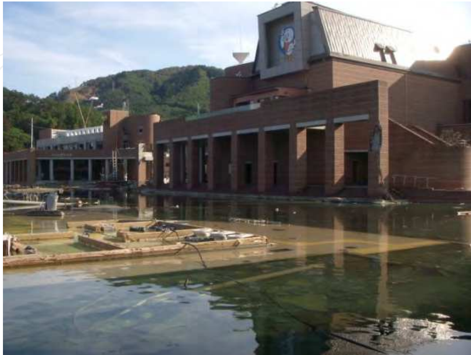
Fig. 33. Waterfront Buildings in Onagawa, Japan Inundated by Tidal Water Due to Earthquake Subsidence. http://tectonics.caltech.edu/slip_history/2011_taiheiyo-oki/index.html
