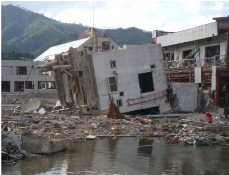
Fig. 38. Overturned Police Station, Onagawa, Japan, 2011.
