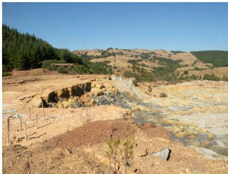
Fig. 24. Upper Scarp of Failed Tailings Impoundment. (GEER 2010)
